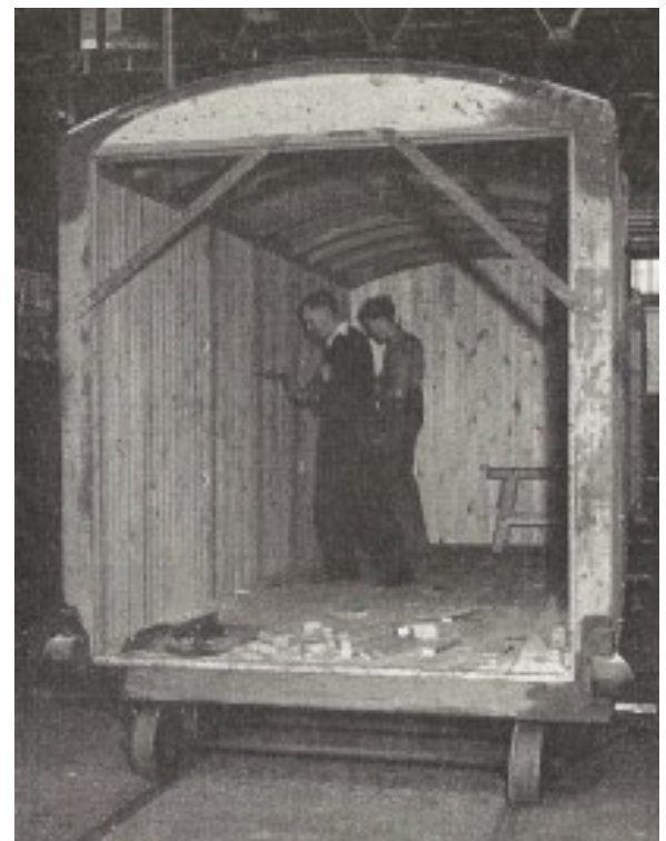
A new BOX B being built at Swindon. The man nearest the camera is fastening the lining using a screwdriver bit in a carpenter's brace, a tool still used in the Teign Valley workshops.
