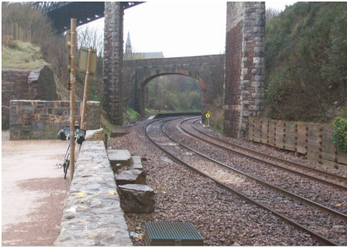
The line turns inland at Teignmouth but still has the Teign estuary to follow. Where the parapet wall finishes was once the eastern portal of East Teignmouth Tunnel, opened out into cutting in 1882.
