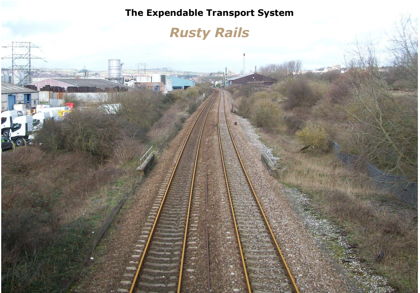
The disused South Devon main line passing beneath Clapperbrook Lane Bridge. Behind the camera is the site of the planned £4-million Marsh Barton Station. Would it have gone 59 days without seeing a passenger train?
