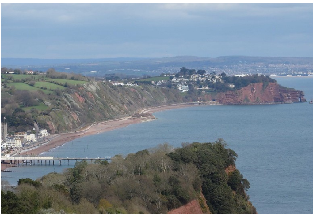
Viewed from the Shaldon to Watcombe road, the whole expanse of cliff towering above the main line can be followed. Part of Holcombe lies above the tunnel mouth, with Hole Head and The Parson and Clerk to the right. Exmouth is in the distance.
