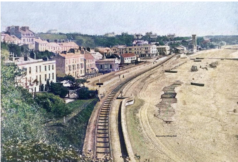
A late nineteenth century view of the broad gauge single line and the 1874 wall, with the seaward face almost covered by the beach. The atmospheric pumphouse chimney can be seen beyond the station.
