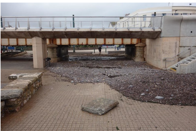
Masonry from the old walls has been used to make seating. One piece of granite has been wrest from its place. The new footbridge now partly blocks the view of Colonnade Viaduct, but it was designed not to be seen from the town.
