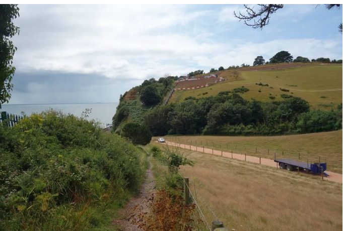
Could this access not have been shared with the tunnel contractor, to save the cost of the scaffolding stairway?
