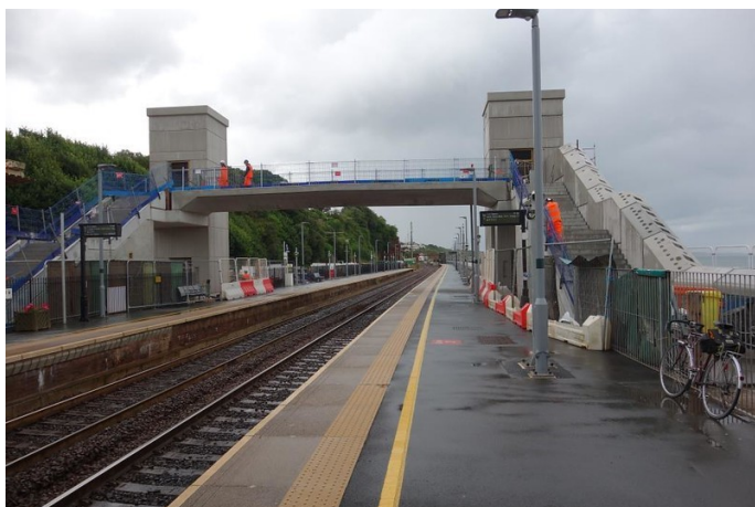
The new, fully-accessible footbridge nears completion in July, 2023.
