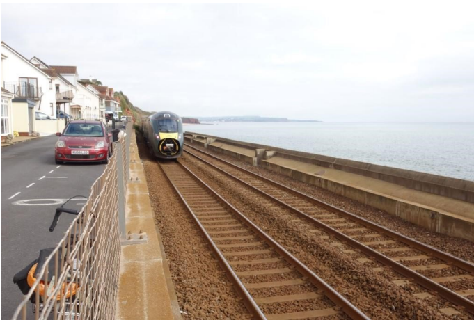
Where engineers stood on the morning of 5th February, 2014, and stared into a gaping chasm crossed by suspended tracks. If the coastline recedes in millennia to come, this 5,000-ton lump of concrete should stay put.
