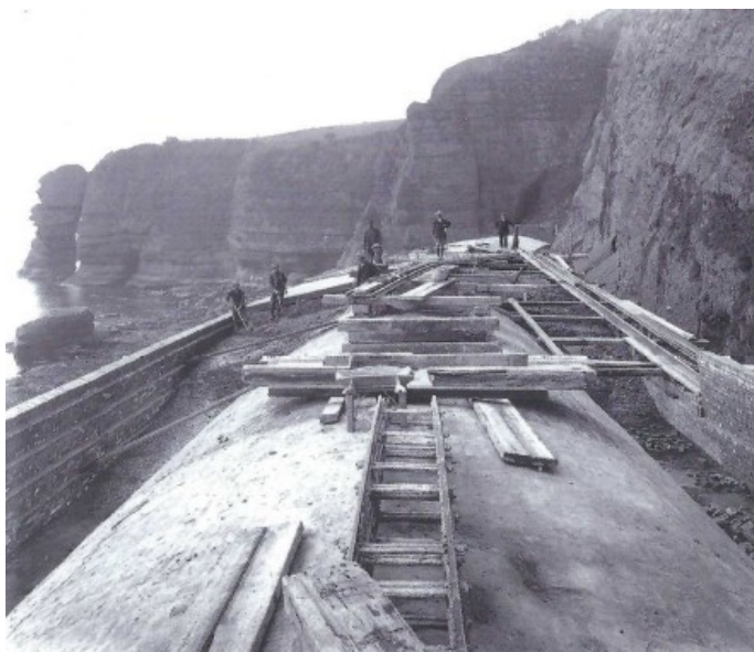
The side walls and crown were completely encapsulated in mass concrete.
