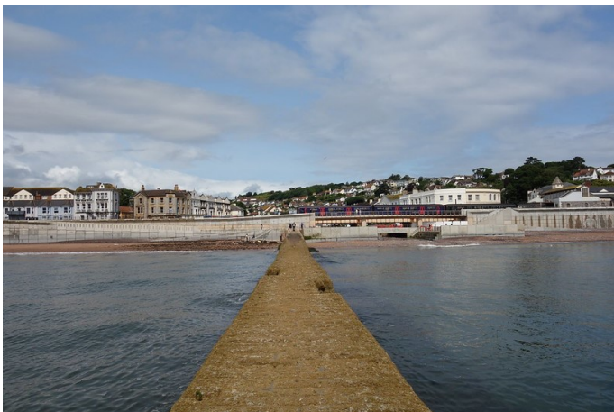
A train crosses Colonnade Viaduct, which appears to be the weakest point of the defensive works.
