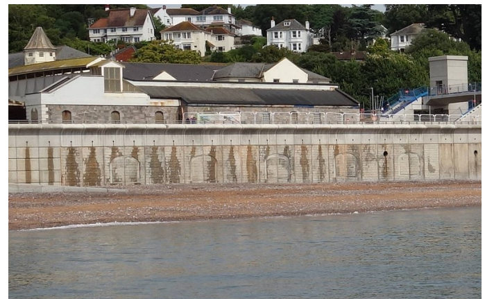
The now buried seating alcoves and masonry of the station building are outlined in what is otherwise a characterless expanse of concrete.
