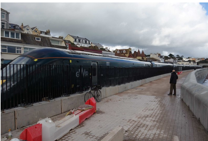
Generations of townsfolk and holidaymakers had watched trains pass above them and had been free to fall off the wall. Now people could look down on the trains and view the sea from behind a thick parapet.
