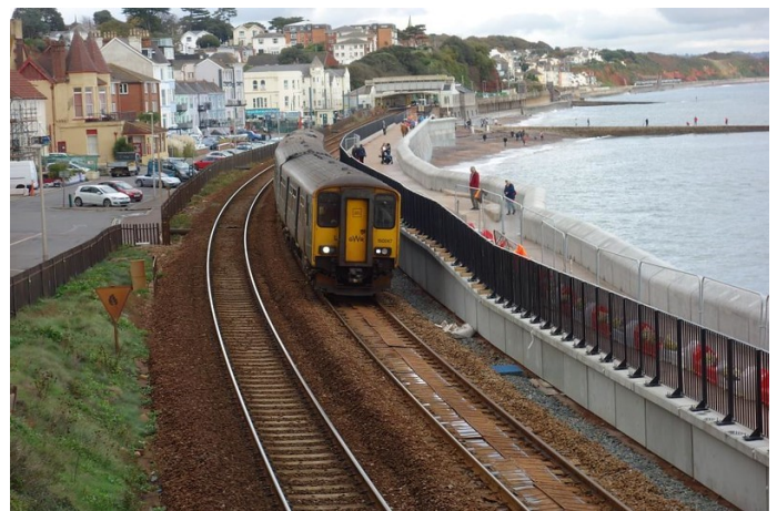
If the sea level rises as predicted, the studies show that much of the 20½ miles between Exeter and Newton Abbot may be vulnerable to inundation. Defending at enormous cost this half-mile length to the point of impregnability may prove in time not to have been the best course.
