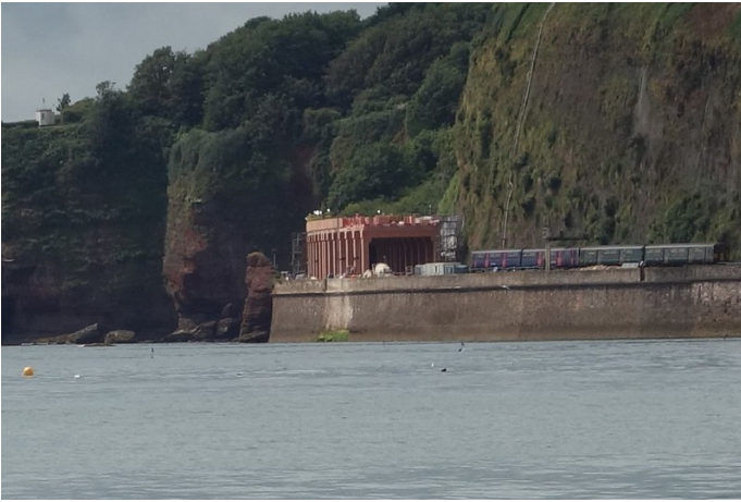
The lightly tinted concrete sections were made by Cornish Concrete in Bissoe, whose yard and works is built on the former Redruth & Chacewater Railway. The sections were brought to Hackney Yard by road, and thence to site by road-rail trailers. The columns rest on piled foundations. The roof will be covered in a yard of sand, both to cushion any large rockfalls and to prevent bounce. The new 120-yard shelter is a continuation of the 147-yard extension of Parson's Tunnel which was completed in 1921.
