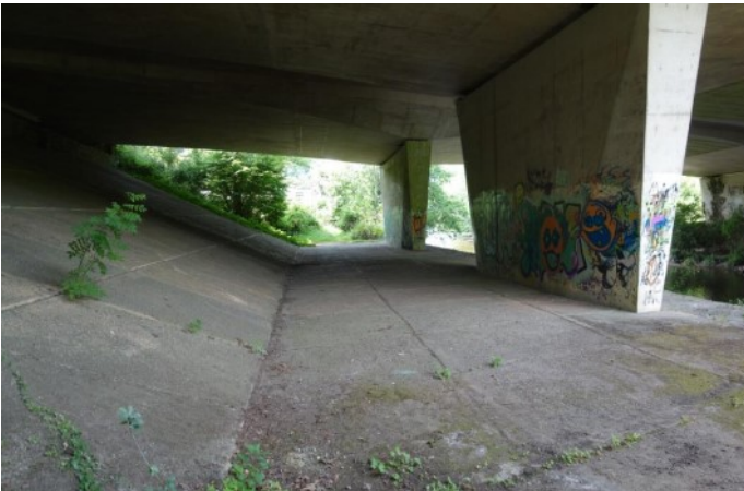
The opening that some imagined could be used to take the railway beneath the road before it bridged the river.
