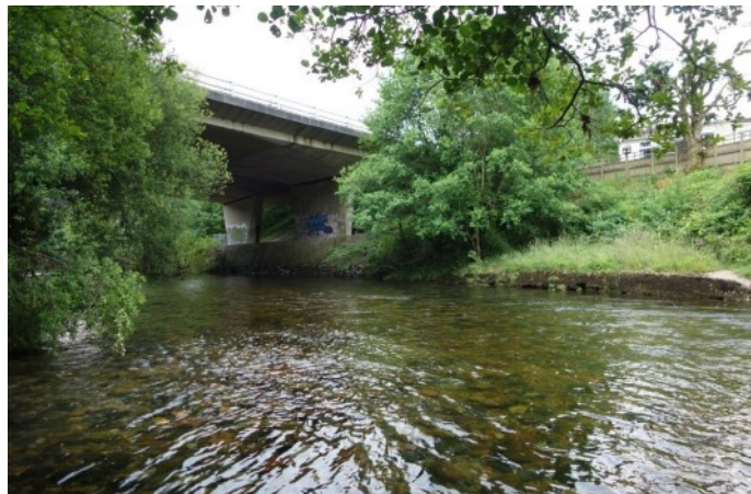
The flood shelf viewed from the opposite bank with the remains of a railway bridge pier at right.
