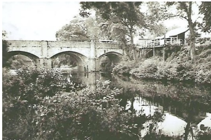
Dart Bridge was built in the 14th or 15th centuries and was widened in the 19th and 20th. The Environment Agency's insistence on a railway bridge being as high and as long as the A38 road bridge ignores the historic restriction just upstream. The railway bridge can just be made out through the left hand arch.
