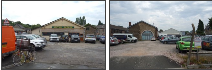
The former Ashburton terminus (left picture) in use as a garage and viewed towards Buckfastleigh. Beyond (right picture) only a few industrial buildings occupy the trackbed, such as the white building next to the old goods shed. Photo 4 May 2013.
