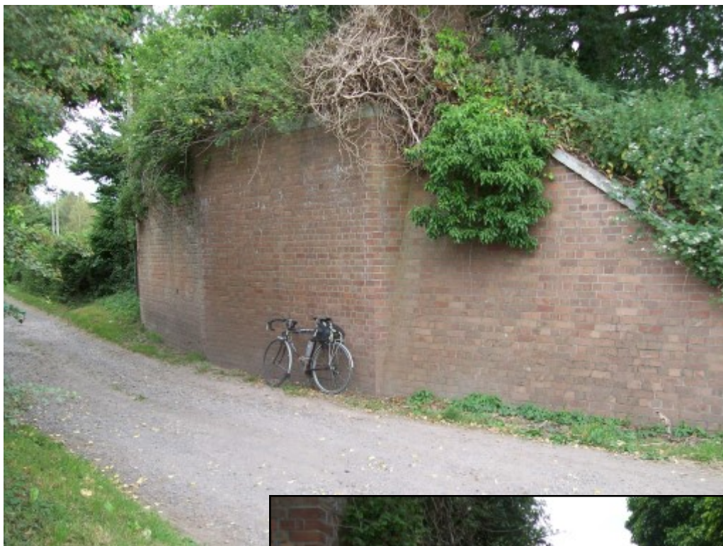
The next bridge , Pontispool, is an occupation, although the lane is also a public footpath. As with Allerford, the “new” work is aligned to the roadway rather than to the original structure.
