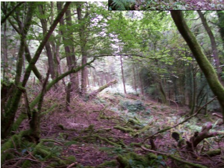
Some rotting fence posts describe the rim of the cutting at the Barnstaple end of Castle Hill Tunnel, although it is hard to see that between the camera and the trees beyond there is actually a large depression.
