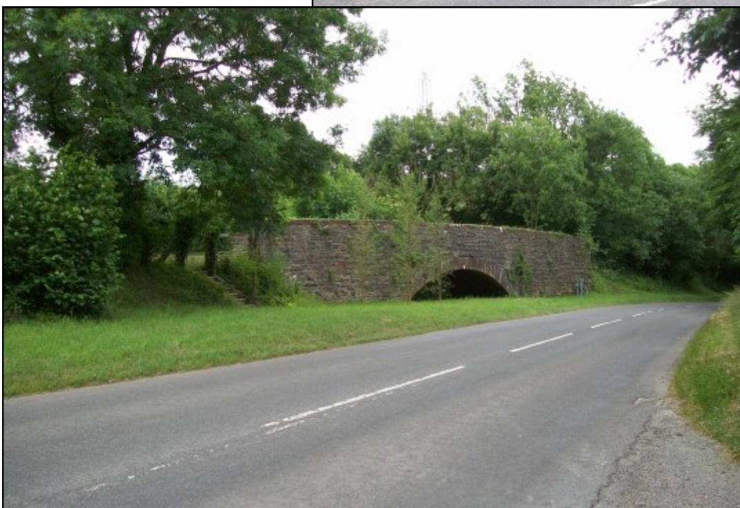
The concrete steps seen to the left of the bridge once led to the signal box and Morebath Junction Halt.
