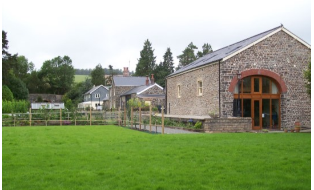
Looking towards Barnstaple from what once would have been the island platform.
