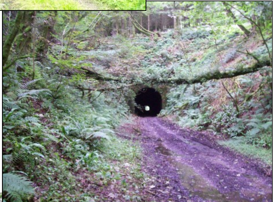
The western portal of Castle Hill Tunnel.
