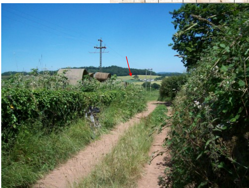
Standing on the now filled-in Quaker's Lane Bridge, not half a mile from Wiveliscombe Station, Castle Bridge can be seen to the left of the twin electricity poles, where the little clump of scots pine stands. My bicycle is leaning against the parapet wall.
