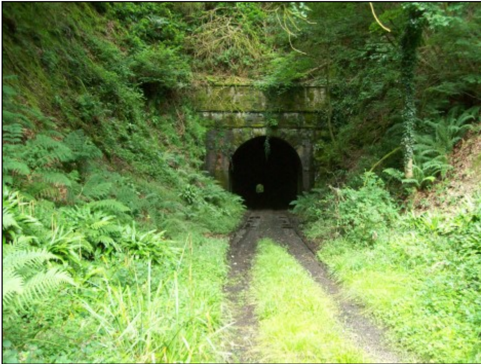
The eastern portal of Castle Hill Tunnel, between South Molton and Filleigh.
