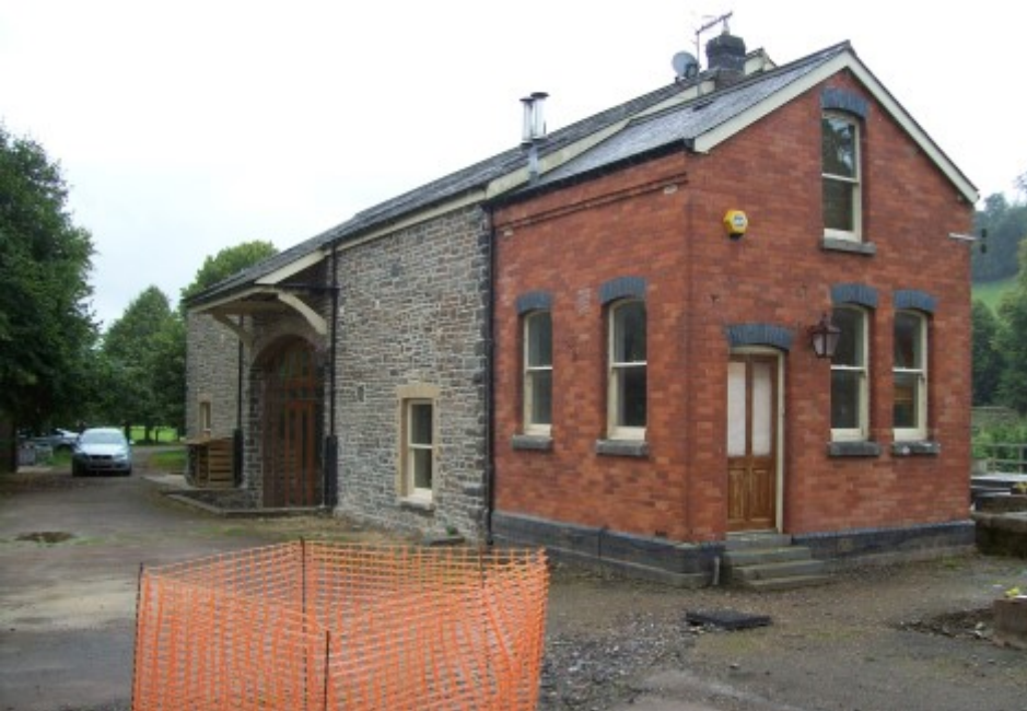
Oddly obscured in two previous shots, the later brick-built extension of the goods shed to provide a large office gives an indication of how much traffic would once have been handled at this railhead on the edge of Exmoor.
