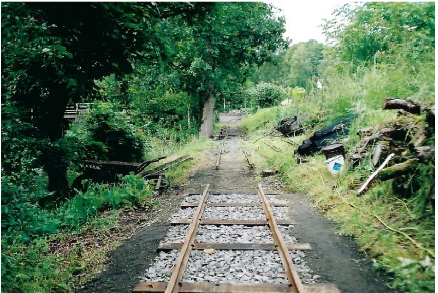
Standard ballast and Meldon crusher dust were used.
