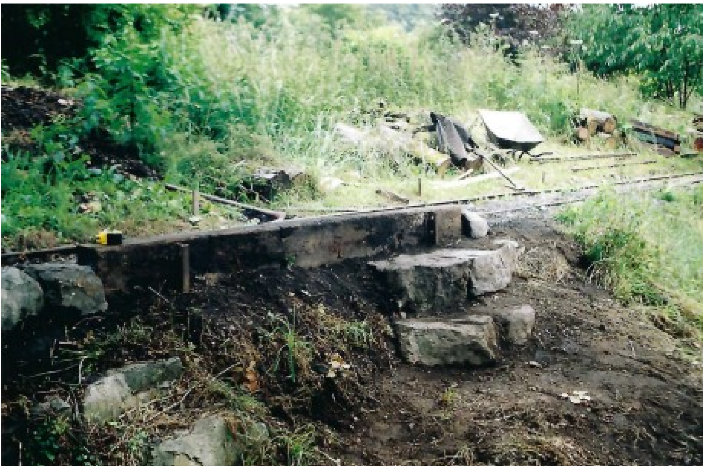
The formation here was retained by a sleeper and made into a feature.
