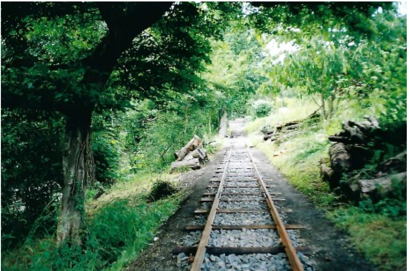
Six new 20 foot, 20 lb. rails were bought for this section. The vertical transitions at either end were done in old 20 lb. 12 foot lengths.
