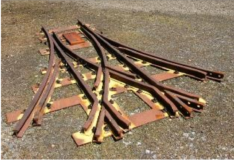
This tandem turnout, or “three-way,” recovered from Balfour Beatty’s railway equipment depot, was overhauled and placed at the top of a short, but severe, incline.
