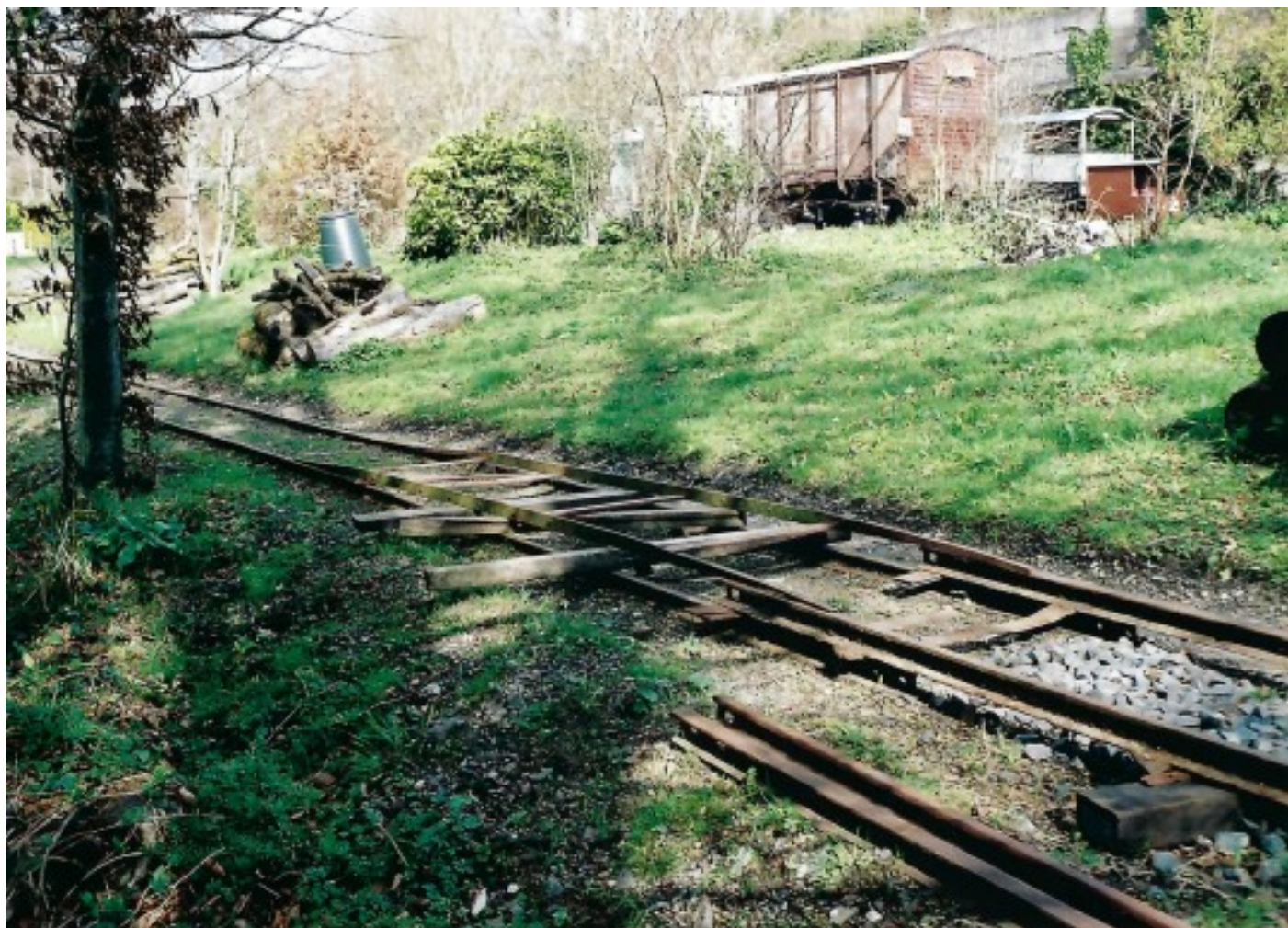
A bridging length was made which allowed movement to continue, albeit very slowly.
