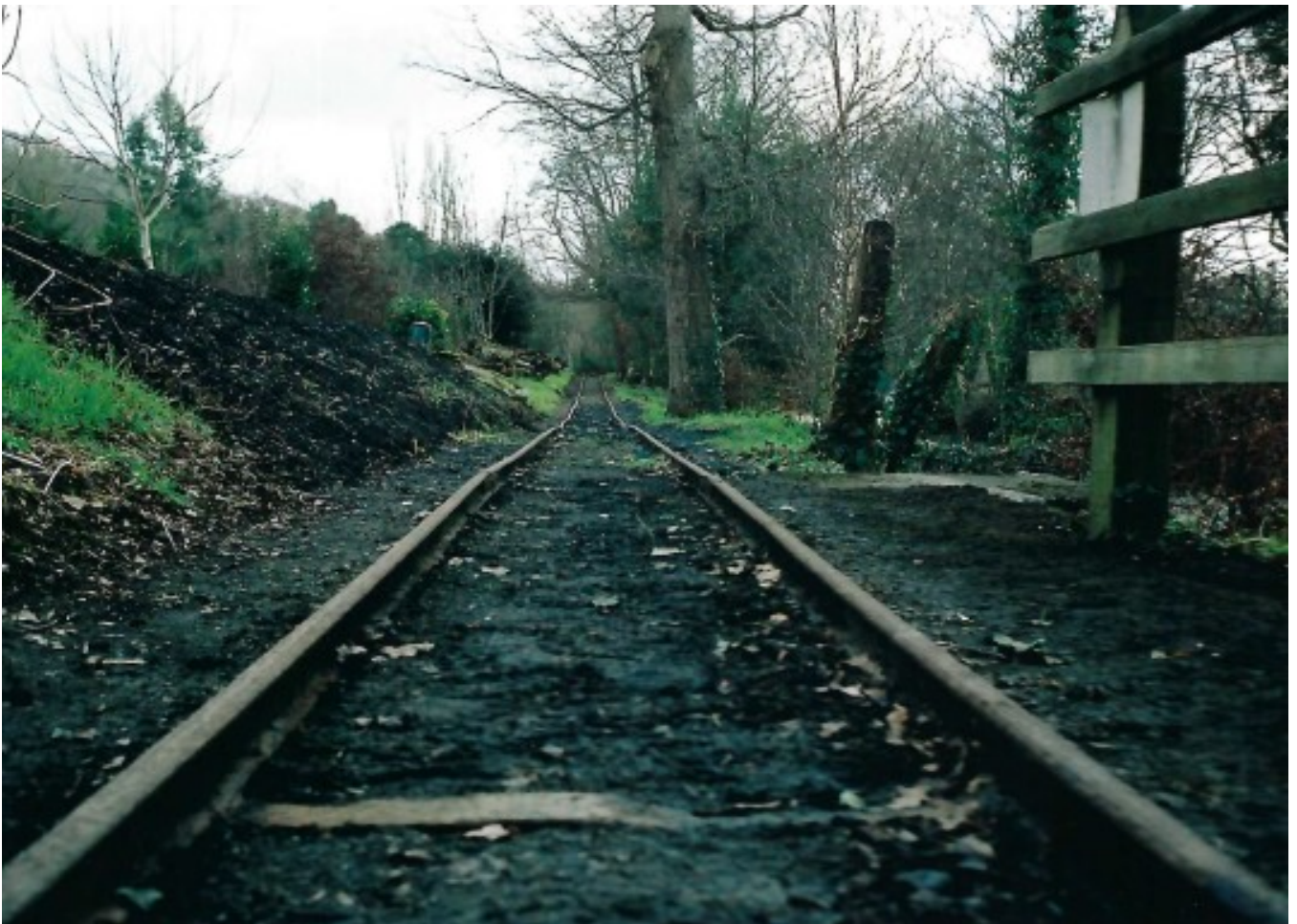
It can be seen that the formation had not been engineered.
