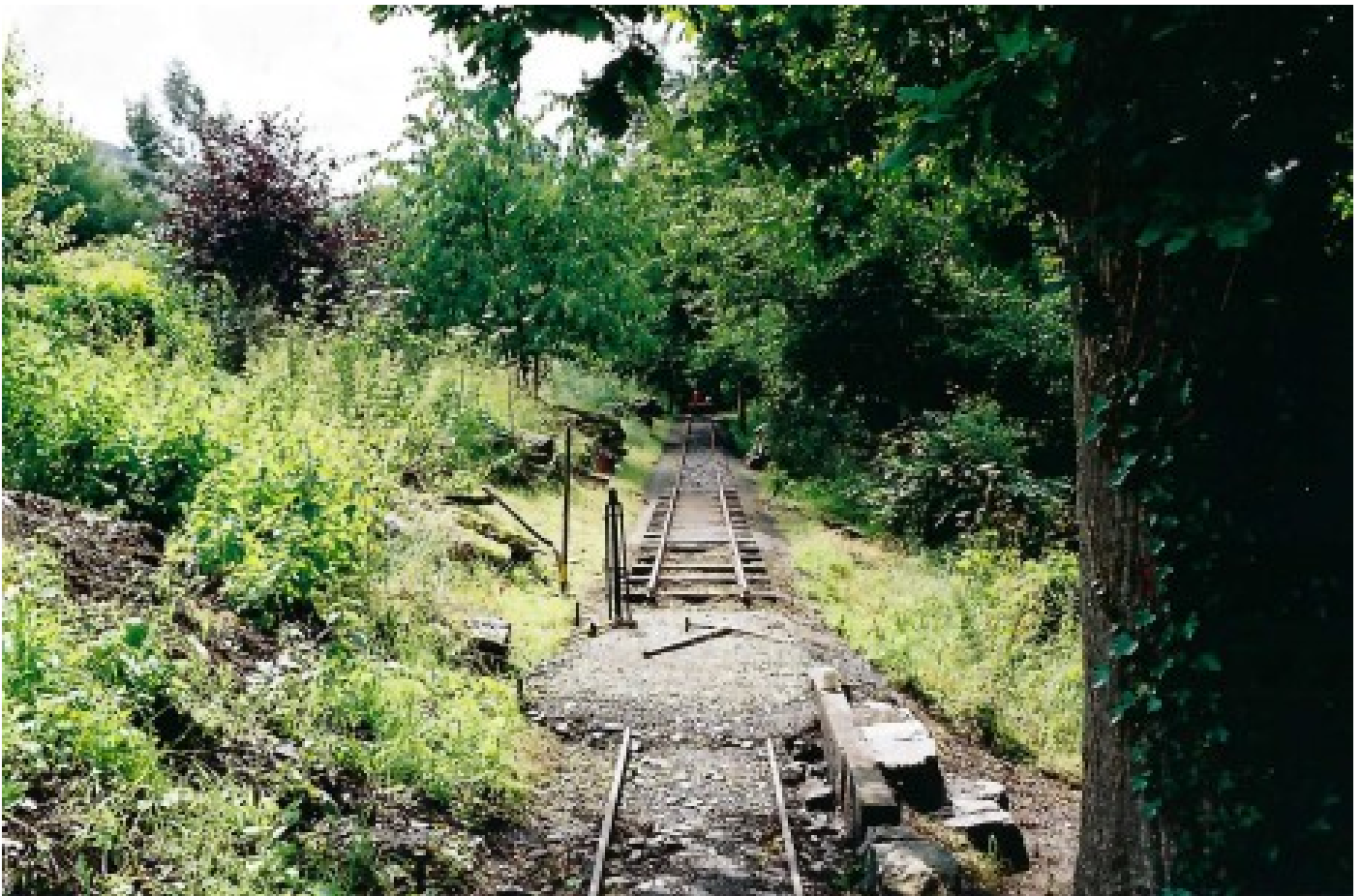
Re-laying is well underway in the summer of 2007. The track had to be raised to make it level. Rails were straightened and spiked to wooden sleepers. "Junction" fishplates had to be made for almost every joint.
