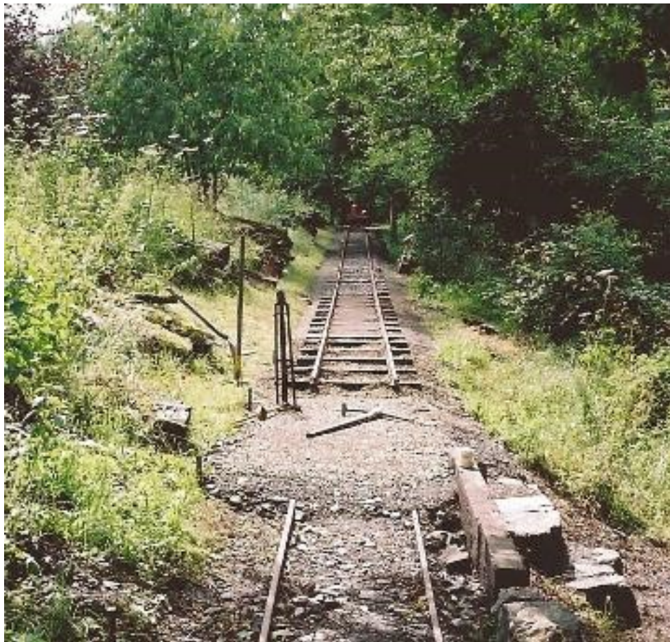
The formation was raised as re-laying progressed.
