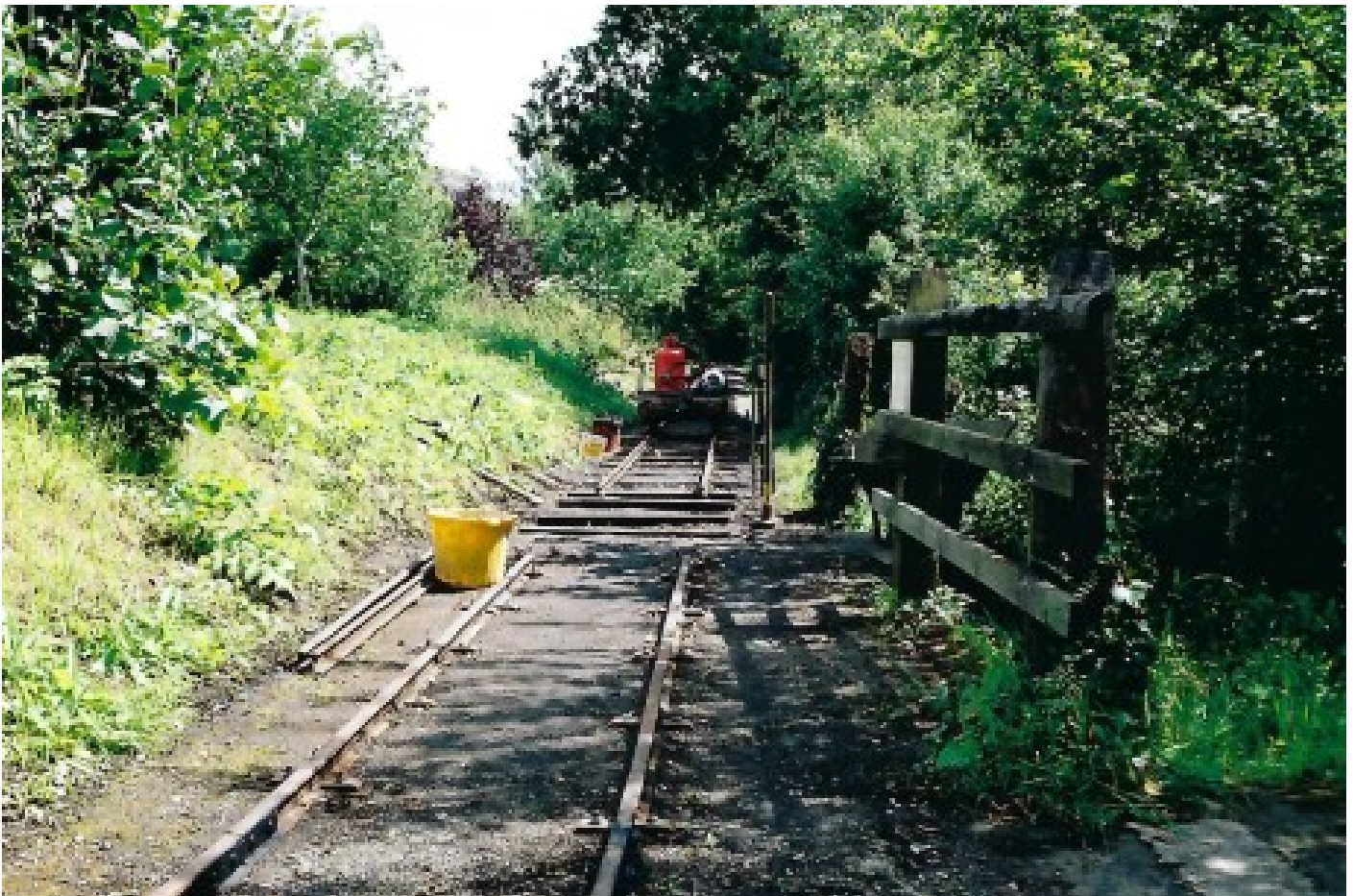
The level was set by the concrete base which had been part of the old ropeway "bridge." The rail fastenings here were chemically anchored to the concrete.
