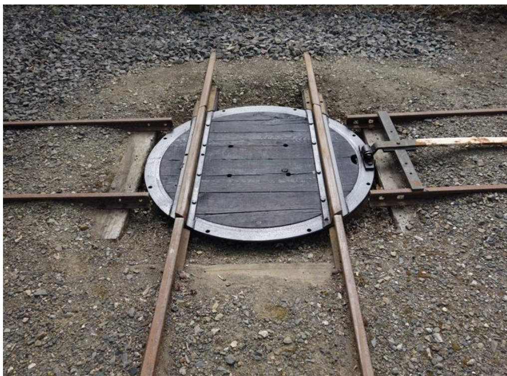
The extension was made possible by the turntable, made from an old lorry turntable trailer.
